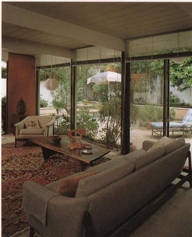
Post-and-beam construction allows for glass panels to abut wooden panels at corner junctions, as seen here. Such construction techniques are inherent in the "pavilion, bringing the outdoors in" design.
